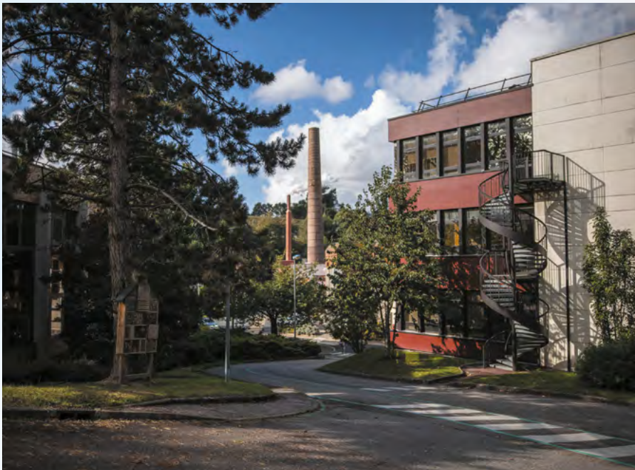
The Oril Industrie facility in Bolbec, Normandy (France).
